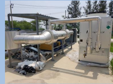
Chiller Heat Exchanger
